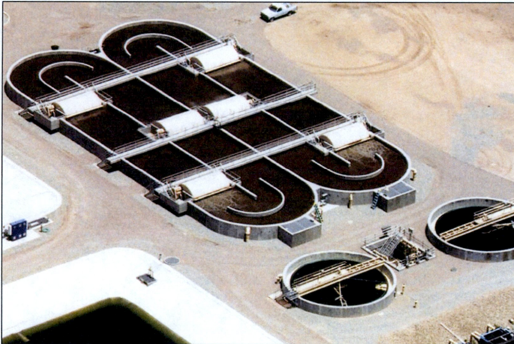
Figure 21.0: Typical CLR Installation with Clarifiers
