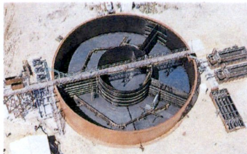
OMNIPAC® SBR Field Erected Package Plant
