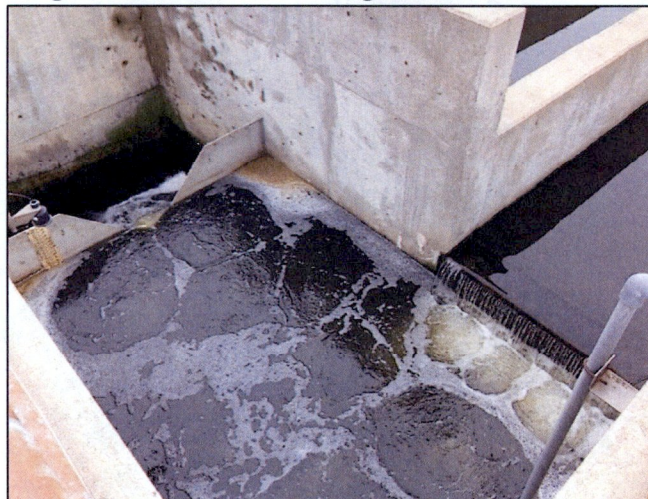
Figure 15.0: Photo of Existing Effluent V-Notch Weir
