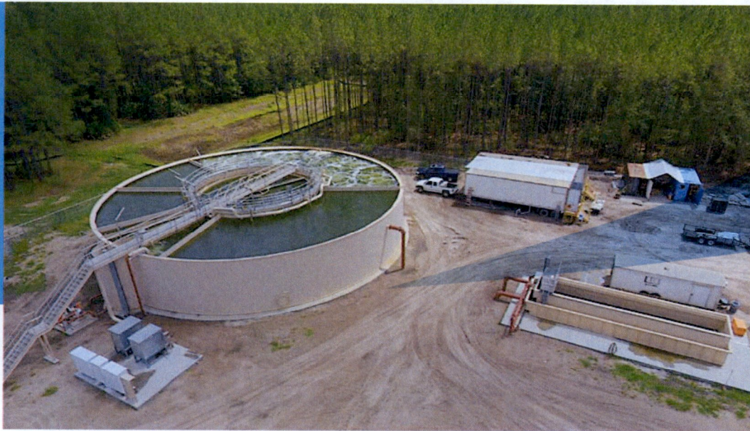
Turnkey Wastewater Treatment Solution in less than six months.
