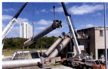
Inspect, repair or replace screw pumps
