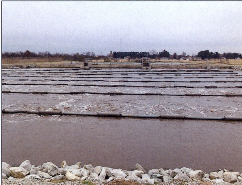
Figure 13.0: Photo of Biolac® System Basin at existing WWTF
