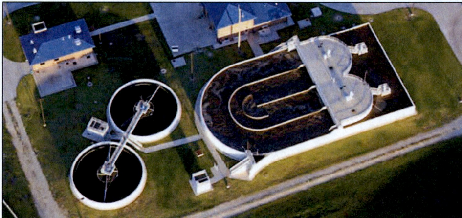
Figure 22.0: Aerial Photo of a WesTech OxyStream™ and COP™ Spiral Blade Clarifier Installation
