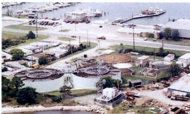
Biological Nutrient Removal Process 1 MGD Installation in Alabama
