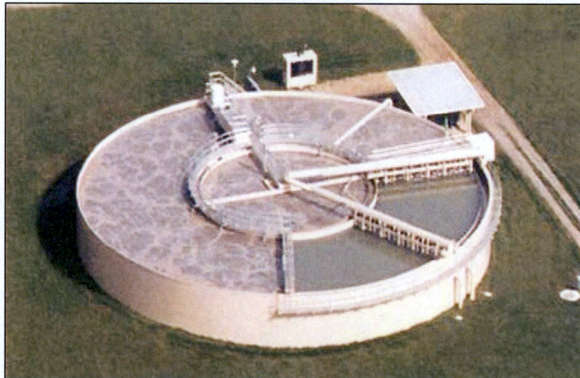
Figure 16.0: Davco Field-Erected System Example, 1MG Dual-Path Process
